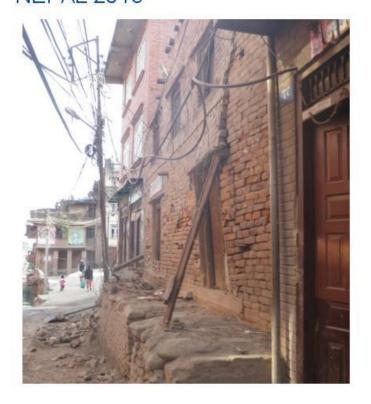
Instabil masonry structures Temporary shored
